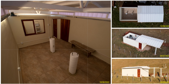
FIGURE 6. The finished observatory.
