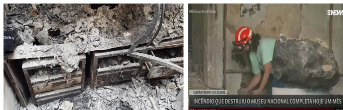
FIGURE 1. Laboratory in which the wooden ceiling burned. The upper floors and ceiling collapsed over the room where most of the meteorite collection was housed.
